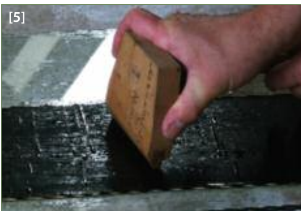
[5] Pushing out the excess glue with a veneer hammer
