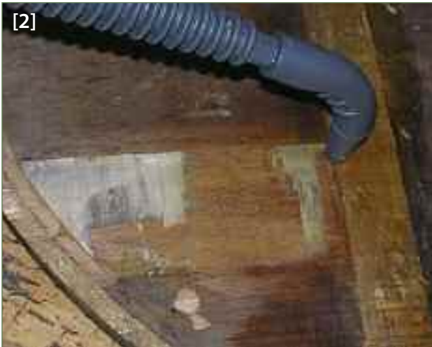
[2] Using the steamer to remove old glue and dirt from the area of the crack
